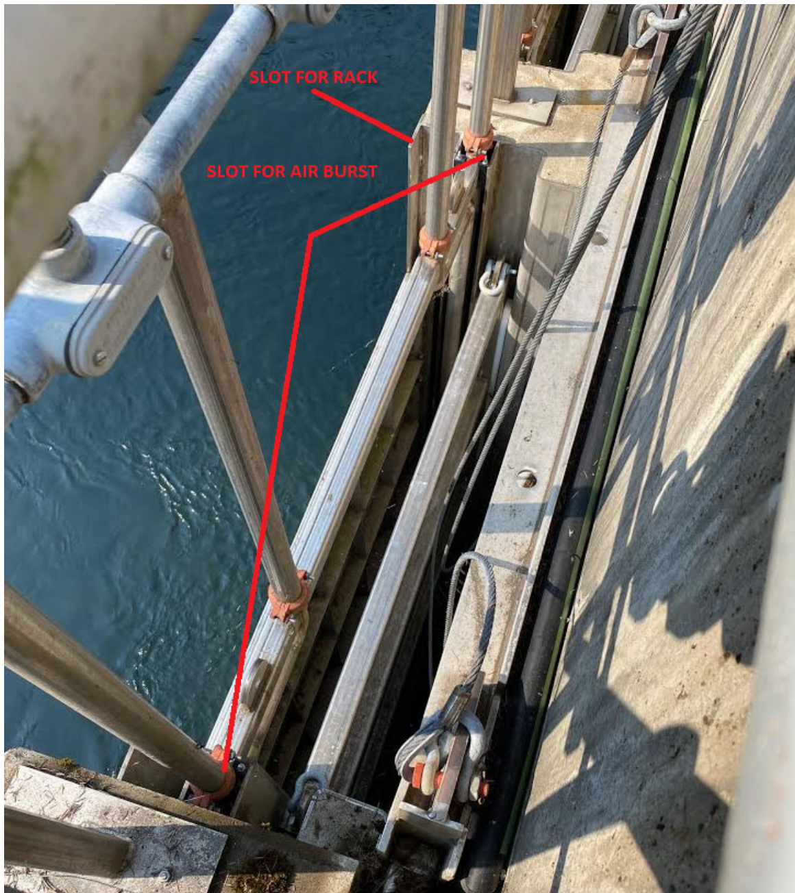
Figure 3-3. Top-down view of Minto Fish Facility air burst, as installed and operating.
